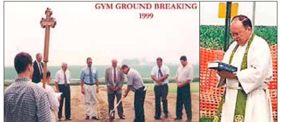
Pastor Block led the groundbreaking service and the Building Committee took the first shovels of soil to break ground.
