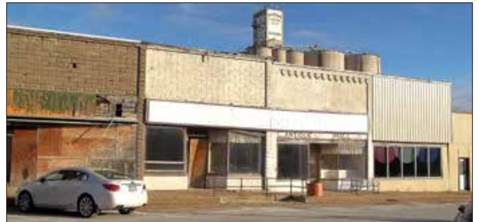
Abandoned buildings on the east side of Main Street
