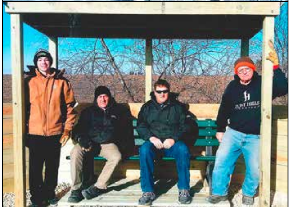
The groundwork and shelter was built by David, Darby, Dallas Wittenburg and Myron Schmidt.
