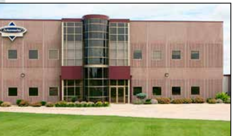
Schumacher's Machine Shop is the original building in Denver, Iowa. Shown above is Schumacher Elevator Company today.
