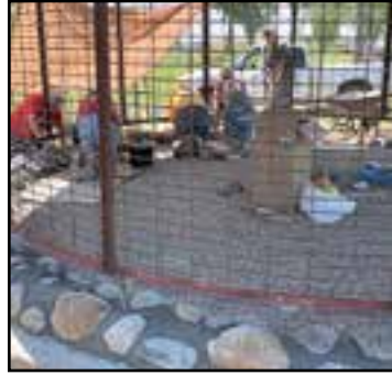
The first rock layer nears completion.
